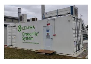
The hydrogen is produced using renewable energy produced by the PV roof installed at Tenova by new high efficiency De Nora's 1MW Dragonfly® electrolyzer, able to supply up to 220 Nm³/h of hydrogen at 30 bar. One of the advantages of this solution is the containerized unit, which allows to minimize civil works (power supply and utilities are already on-board), proving the
